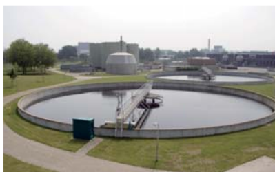
Waste water treatment
