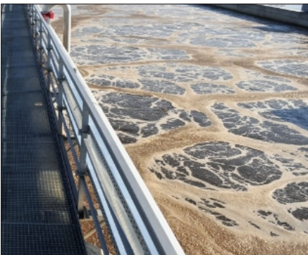
Wastewater Treatment Power Generation
